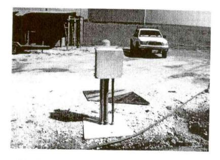
View of one of four junction boxes for leak detection and cathodic protection systems.
