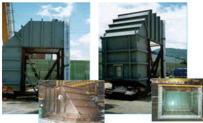
Figure 35. Frame 7E plenum during installation.
