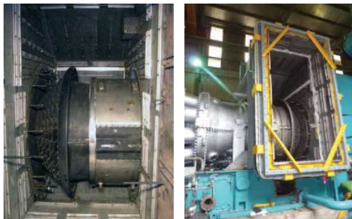
Figure 36. Installed 6B plenum and exhaust frame assembly.
