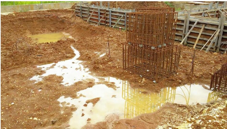
10) July 12, 2018 at Talofofo (Overnight rain / Can not proceed compaction work)
