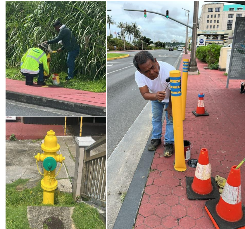
Repainting of Fire Hydrants & Bollards
